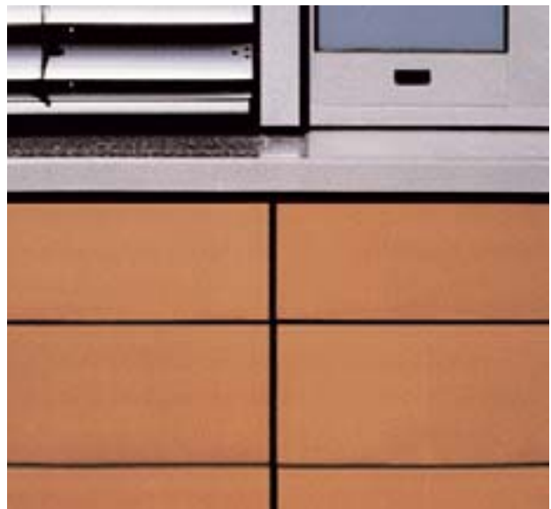
TILE FAÇADE WITH CLASSIC EXTRUDED PROFILE AND CONNECTION TO THE WINDOW-LEDGE
